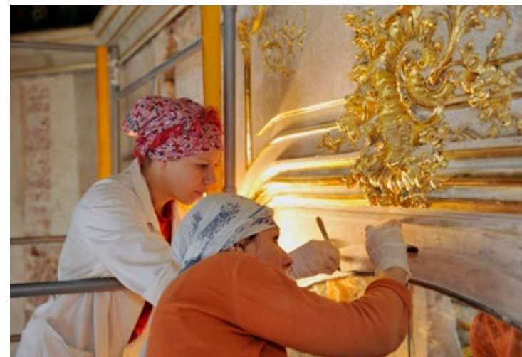
Conservation works in the Wilanów Palace, photo W. Holnicki
